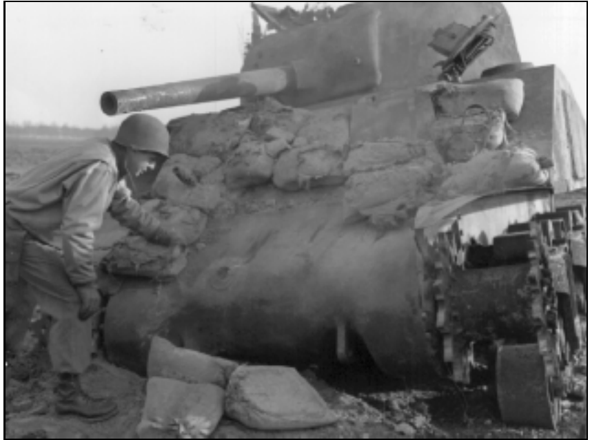
Testing ways to improve the Sherman's protection, units fired captured German antitank weapons against hulks. Above, a soldier examines the damage done by a 60mm shaped charge that blew away bags of cement before perforating the transmission casting. Spare track sections were also employed, as seen on the Sherman below, at the 1st AD's crossing of the Arno River in Italy during 1944.
